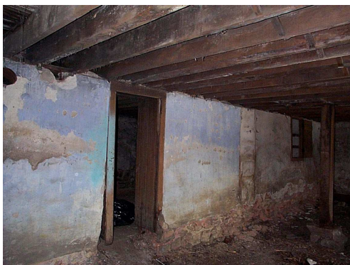
Pictured left is the full 18 inch thick center wall discovered in the basement during the cleanout phase.
